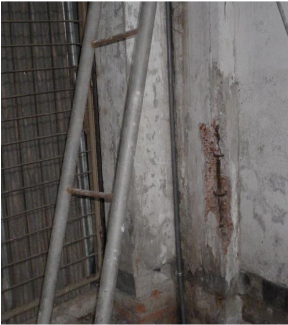
Photo-1: column before retrofitting
