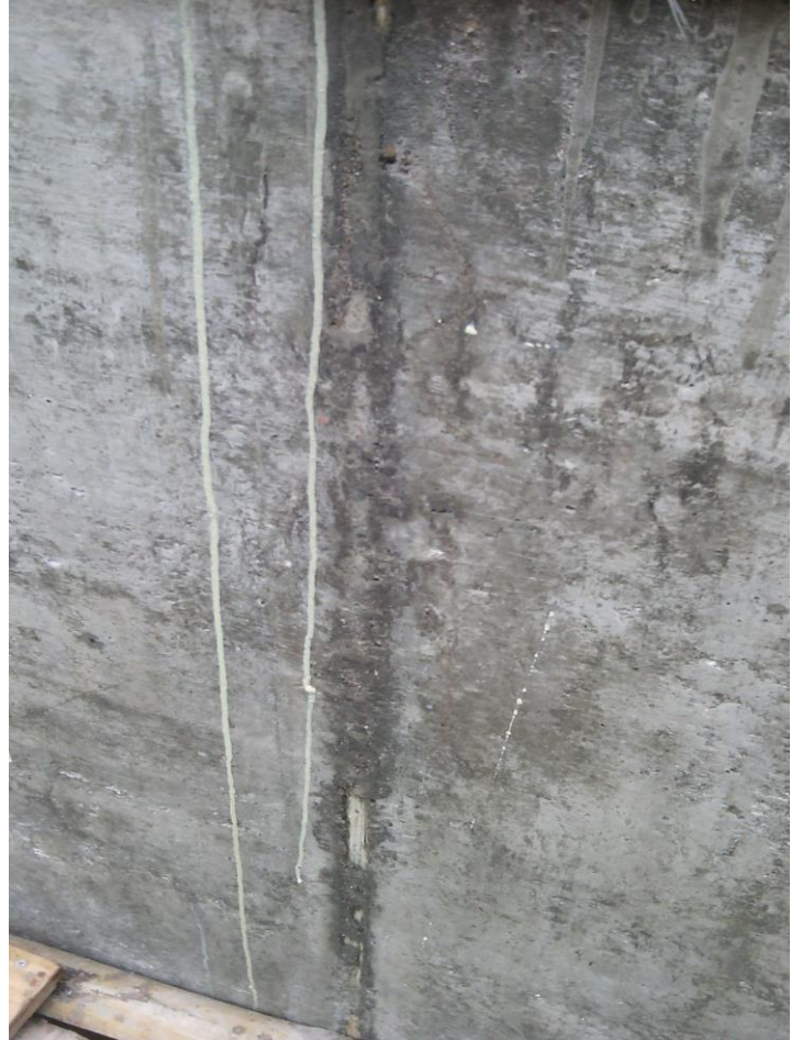
Photo-6: Column after retrofitting
