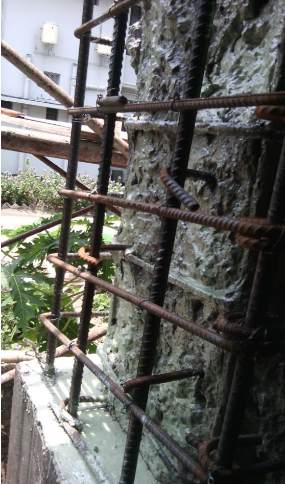
Photo-5: Column During Retrofitting
