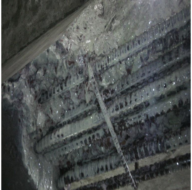
Photo-2: Cracked Section of Beams
