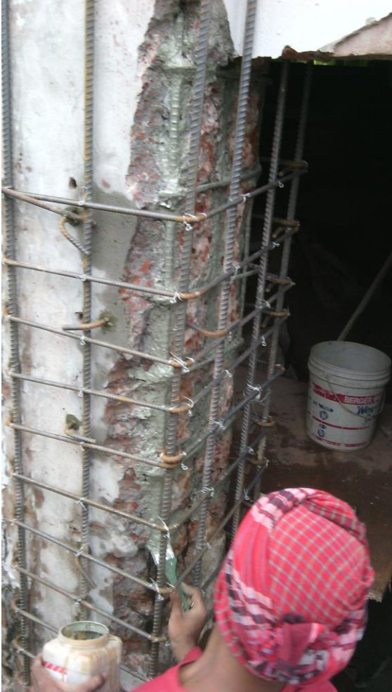
Photo-3: Columns During Retrofitting
